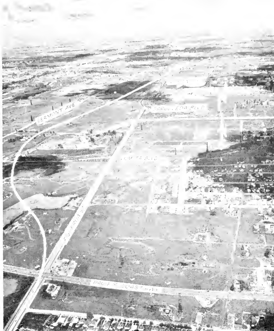
Looking northerly along Harbor Freeway route, showing Los Angeles downtown area background right, Los Angeles County Sanitation Plant shown center left
